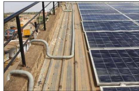
No Cable tray provided! Cables enclosed in PVC Pipes
