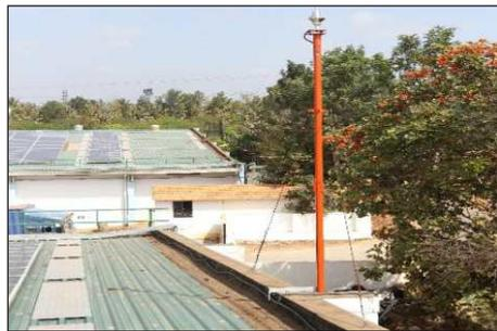
Lightening Arrestor ( ESE type) Covering 105 mtrs radius
