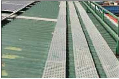
AC Cable trays provided to walk on, as well as prevent wiring from being damaged
