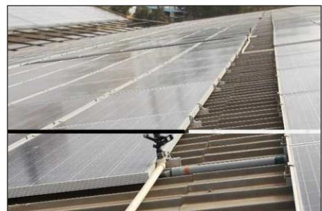
Small sprinklers are used which leads to poor panel cleaning
