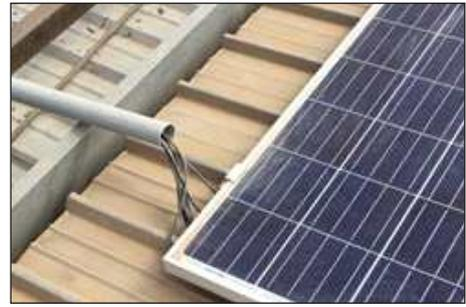
Exposed wiring will get damaged and is also dangerous
