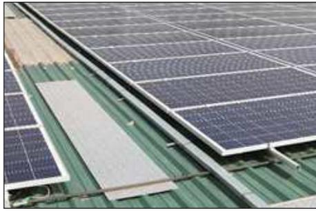
Well enclosed wiring in DC Cable tray
