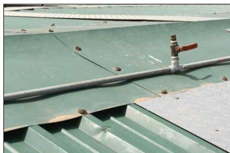
Panels are cleaned using Pressurized pump with GI pipe
